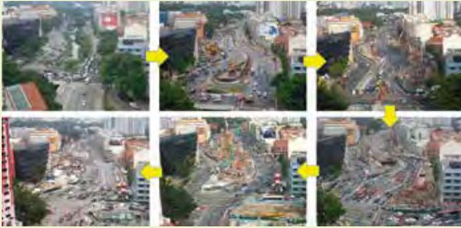
Construction of the Downtown Line Rochor Station under the busy Bukit Timah Road and existing Bukit Timah Canal required diversion of the canal and multiple stages of temporary road and traffic diversions that involved close coordination and interfaces with numerous stakeholders such as utility companies, government departments, building owners etc.
