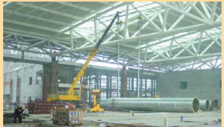
Installation of exhibition hall aircon ducts
