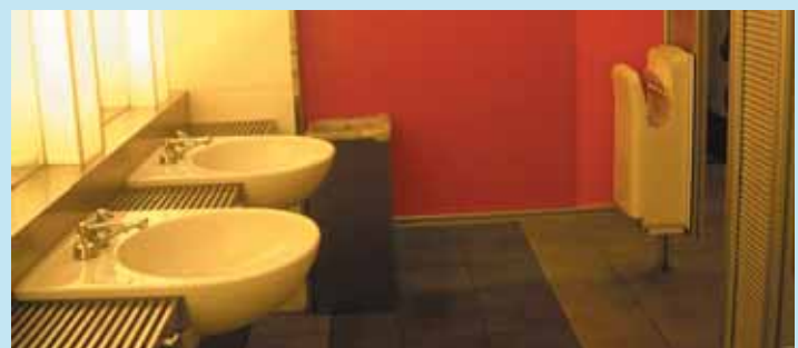
Toilets with user-friendly basin counters equipped with hooks for shopping bags, and energy saving hand dryer
