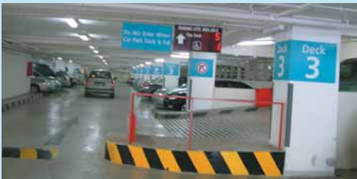
Brightly lit carpark with parking guidance system to lead motorists to available lots
