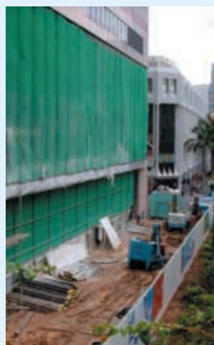
Upgrading of facade
