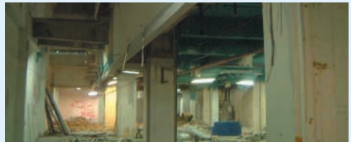
Reconfiguration of interior layout and M&E works
